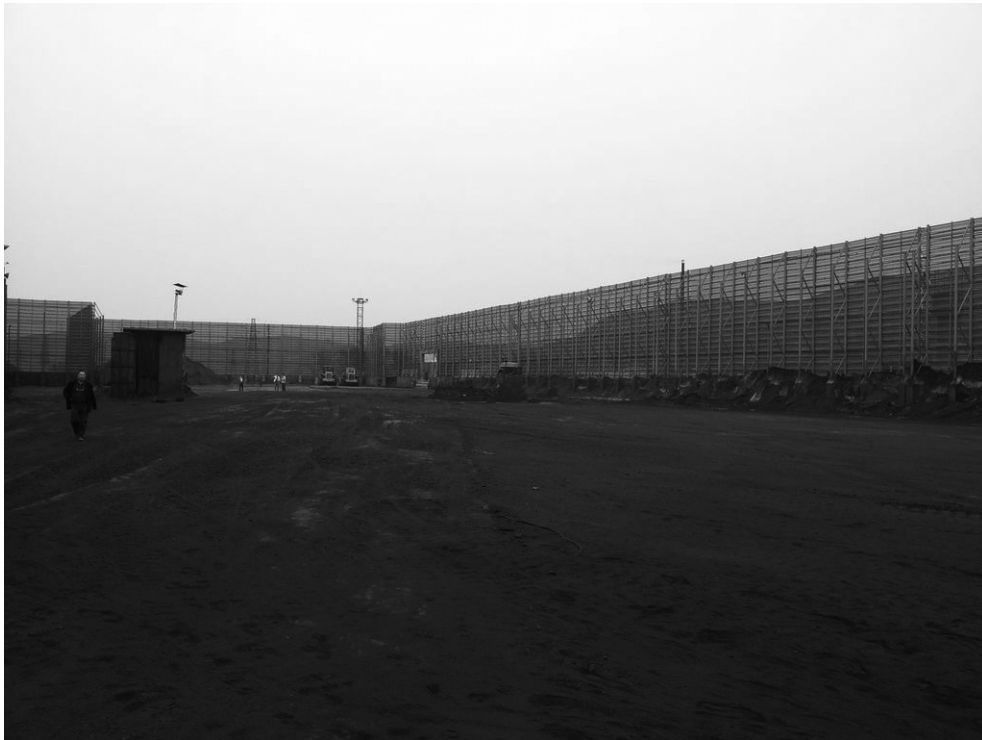
Coal storage compound with reduced dust emission fencing (Not owned by the Target Company)
