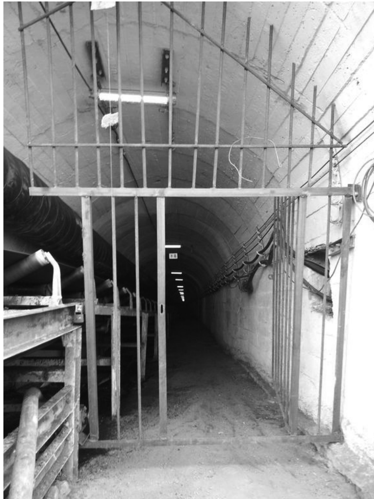
Coal conveyor incline at Jinxin Mine, looking down the incline
